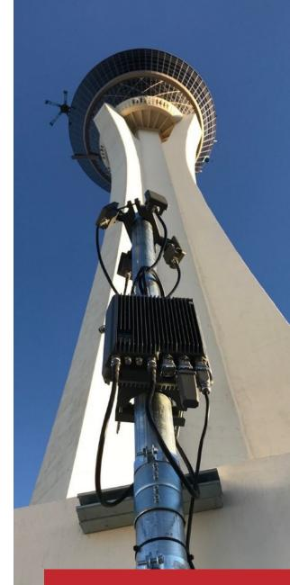
Aeroscrope RF Sensor
